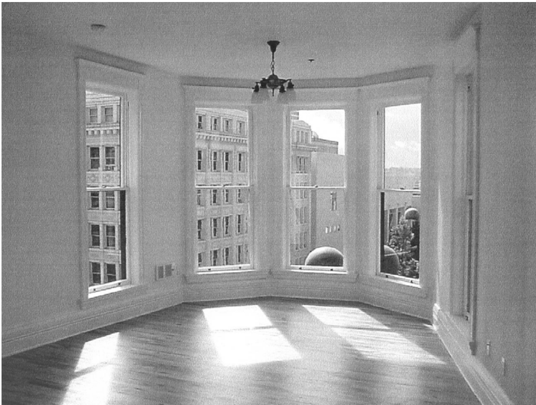
Bostwick 6.14: The apartment units feature large repaired historic windows, as well as historic trim and wood floors.
