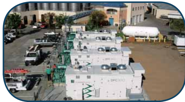
Sierra Nevada Brewery, Chico, California. Alliance Power Inc. worked with the Sierra Nevada Brewery to install a 1-megawatt CHP system operating since 2005 with four 250-kilowatt Direct FuelCell® high-temperature molten carbonate fuel cells. The CHP system provides nearly 100 percent of the facility's base load power while waste heat is used as steam for the brewing process and for onsite heating.
