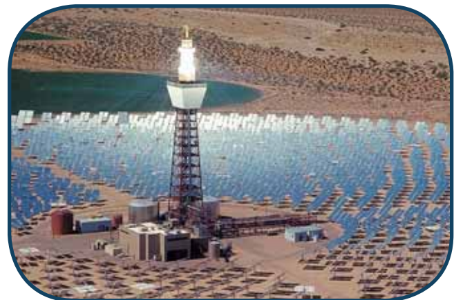
Solar Two's power plant heliostats focus sunlight onto the central tower receiver, providing a clean, renewable source of energy.
