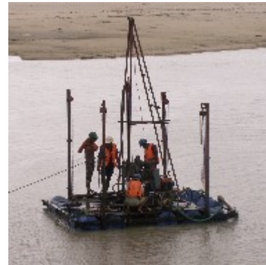
Geotechnical drilling in Arugam Bay in preparation for a detailed design of the new bridge
