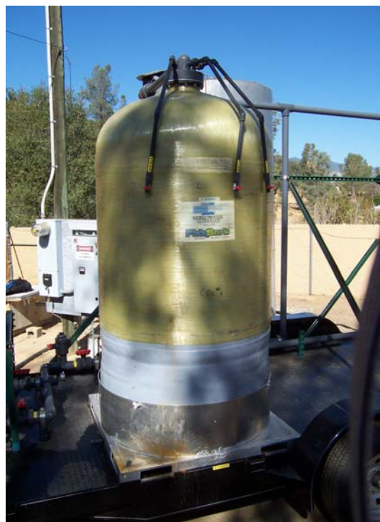
Figure 4-7. HIX Media Vessel with Pressure Release Port and Media Sampling Ports
