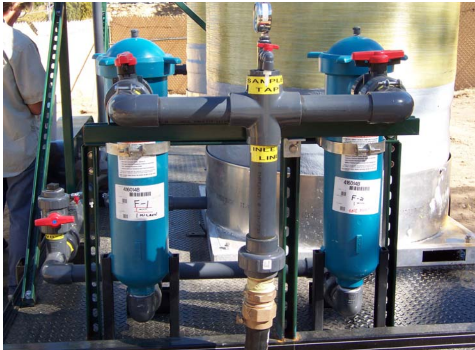
Figure 4-6. Bag Filter Assemblies
