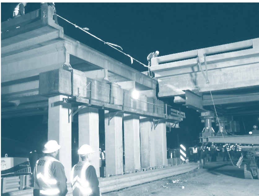
Figure 10. Installation of LaDOTD I-10/LA35 bridge.
