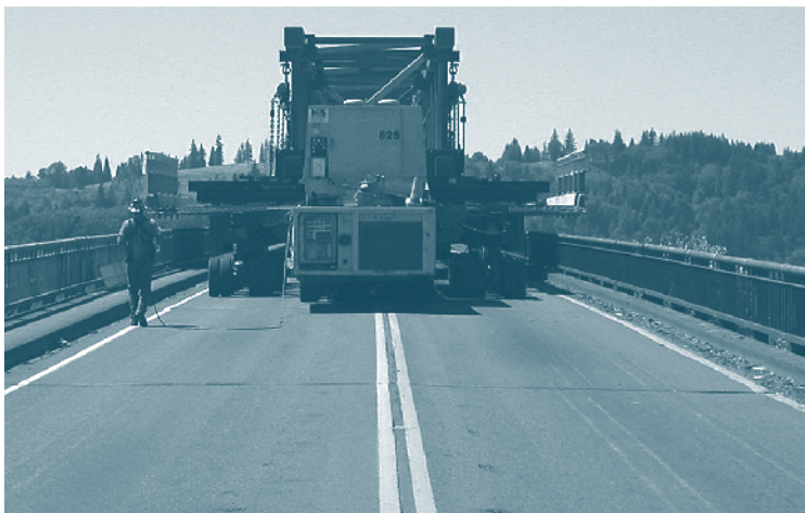
Figure 13. WSDOT Lewis and Clark bridge deck replacement.
