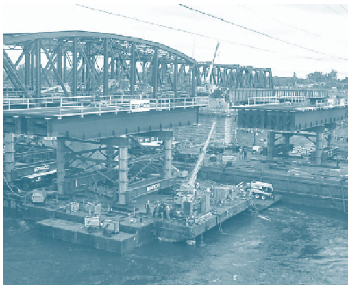
Figure 2(a). Titan Bridge Lift System.
