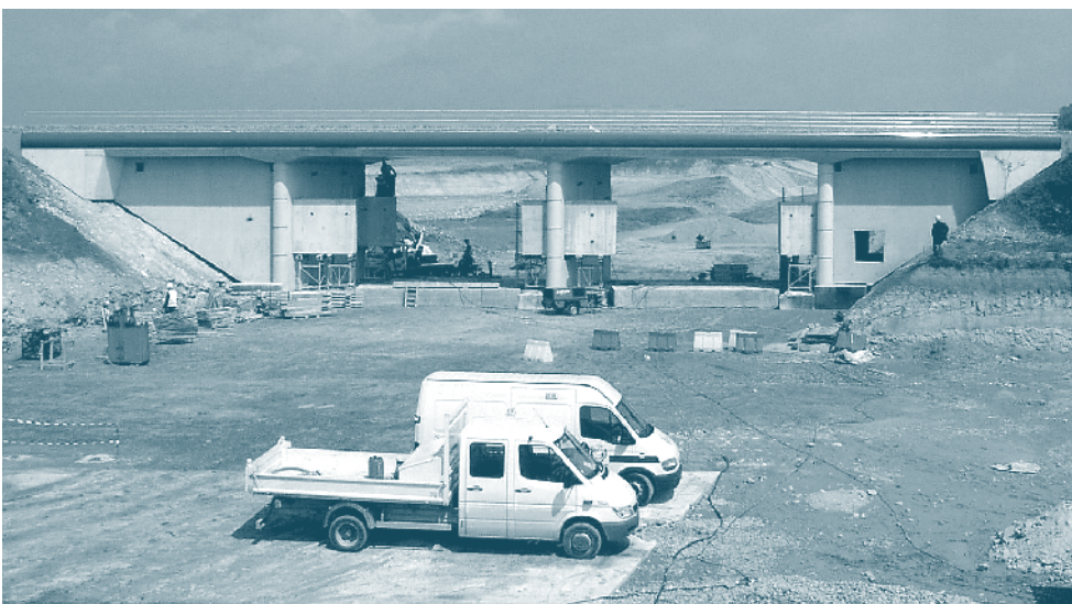
Figure 15. SPMTs moved four-span PRA 1309 railway bridge in France.
