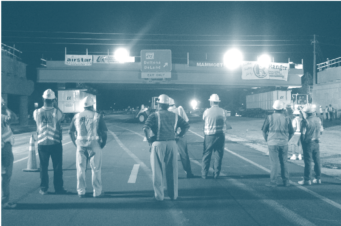
Figure 9. Installation of FDOT I-4 East Graves Avenue bridge.
