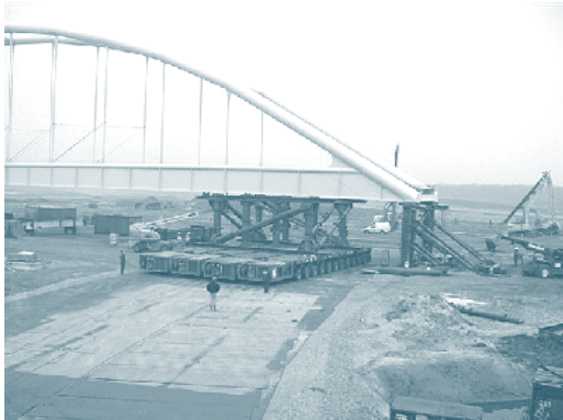
Figure 3. Substructure for temporary bridge support for Nootdorp Bridge in the Netherlands.
