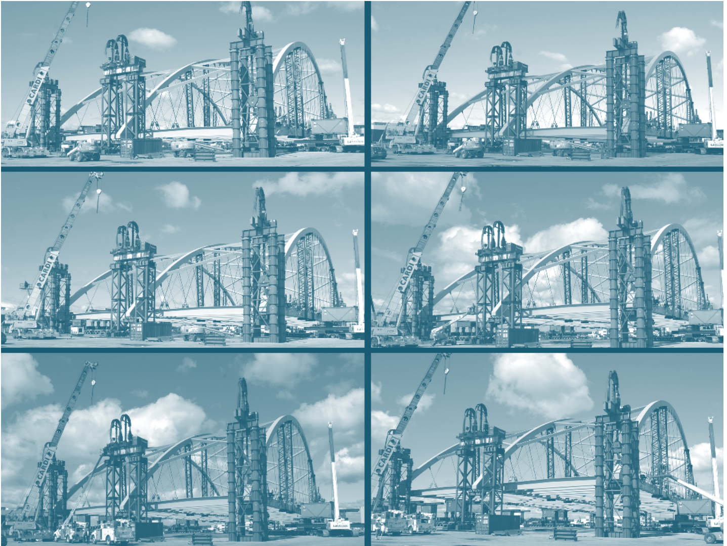
Figure 2(d). Strand jack system.
