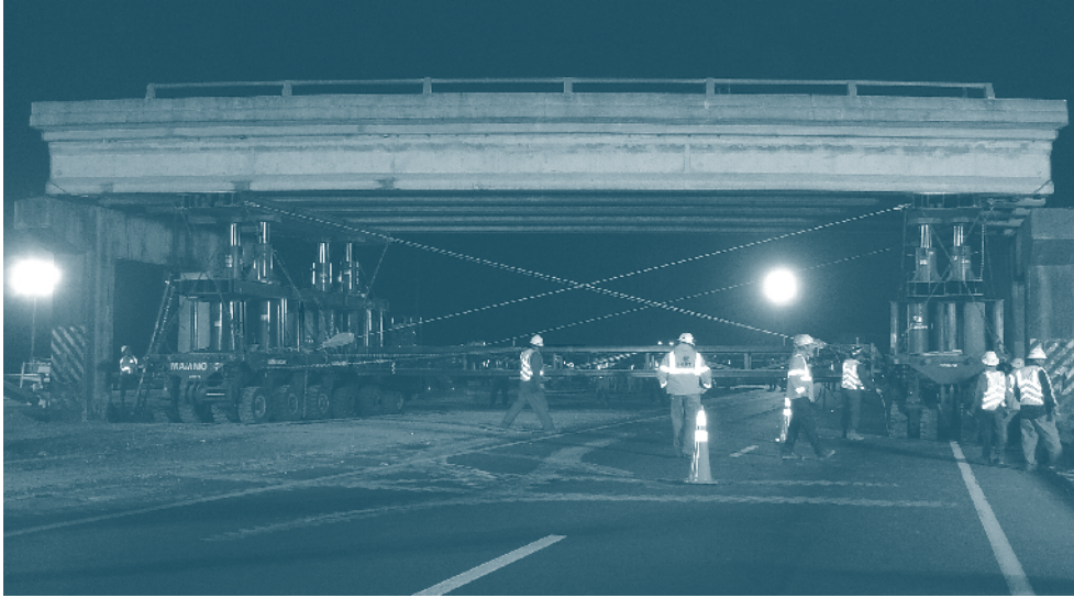
Figure 8. Removal of FDOT I-4 West Graves Avenue bridge.
