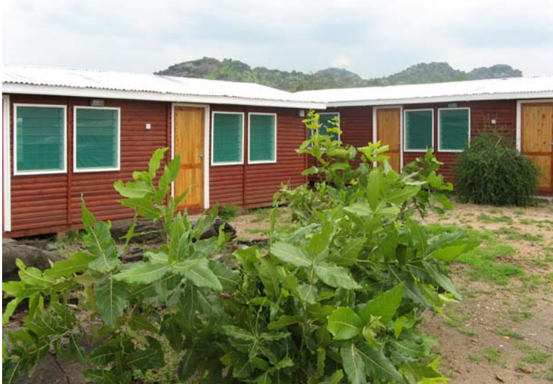
New office buildings enhance the Southern Sudan AIDS Commission's capacity to coordinate a multi-sector response to HIV/AIDS.
