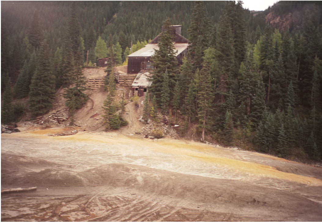
Figure 6. Yellow and gray tailings from Lackawanna Mill (site # 287) were placed in flood plain of the upper Animas River, east of Silverton. Because of evidence that the tailings were releasing contaminants to the river, the BLM removed the tailings in 2001 and emplaced them in a repository at the May Day mine.
