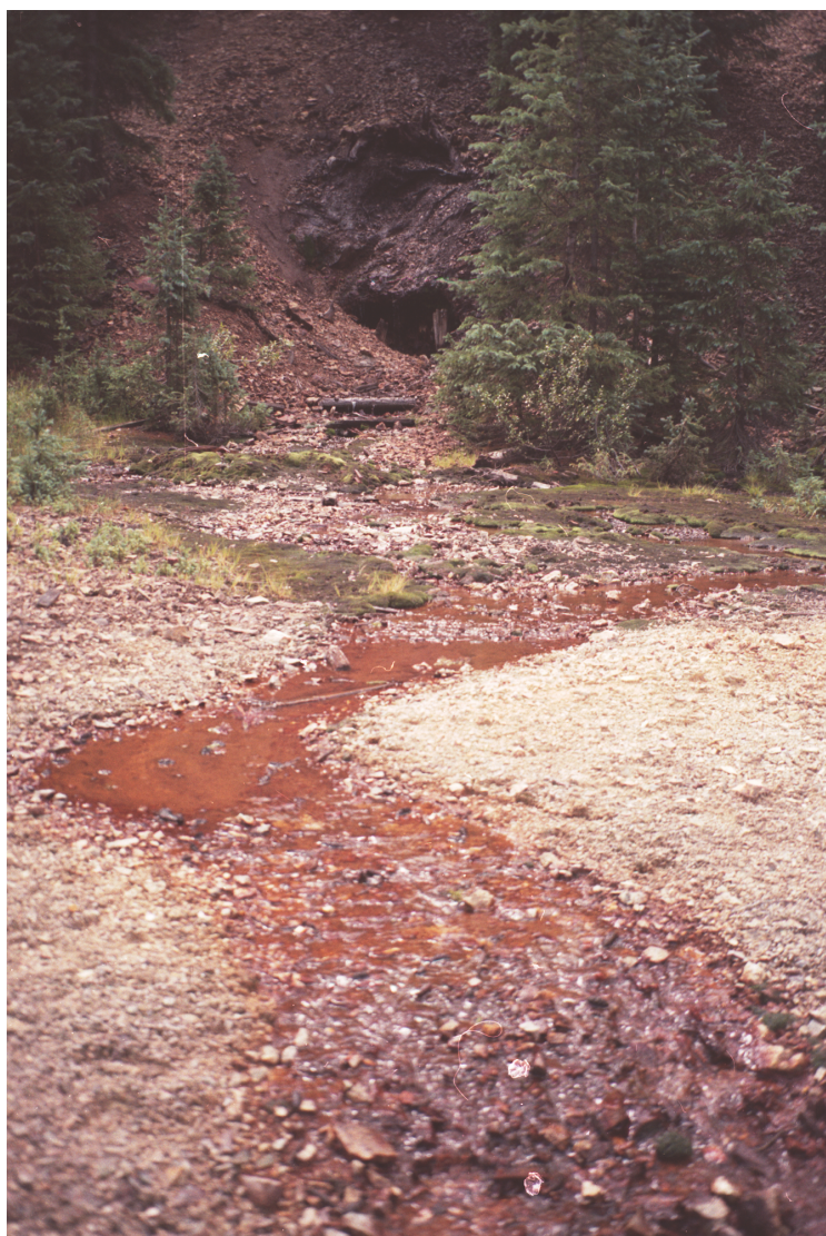
Figure 19. Lower adit of Bonner mine, and drainage discharge that flows to Middle Fork Mineral Creek.
