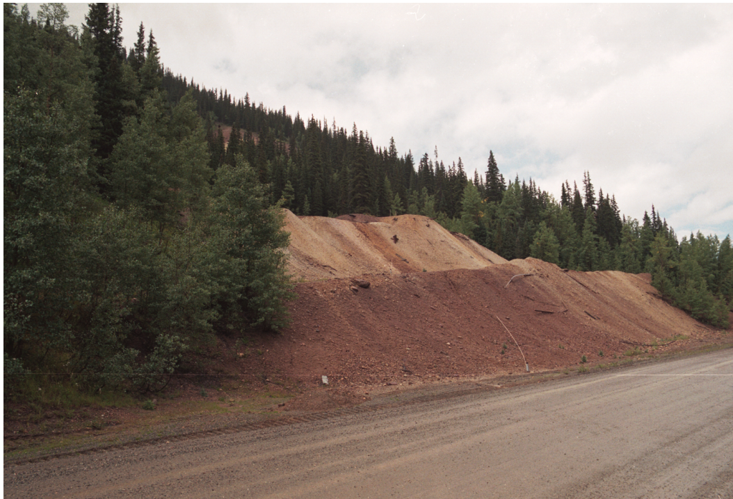
Figure 12. May Day mine, excavated to explore veins west of Cement Creek, created these large waste piles of sulfidic rock. To minimize reactions from snowmelt and rain, the BLM reclaimed the dump in 2001 by emplacing a geosynthetic liner and covering with clean soil. Lackawanna Mill tailings were also emplaced there at that time.
