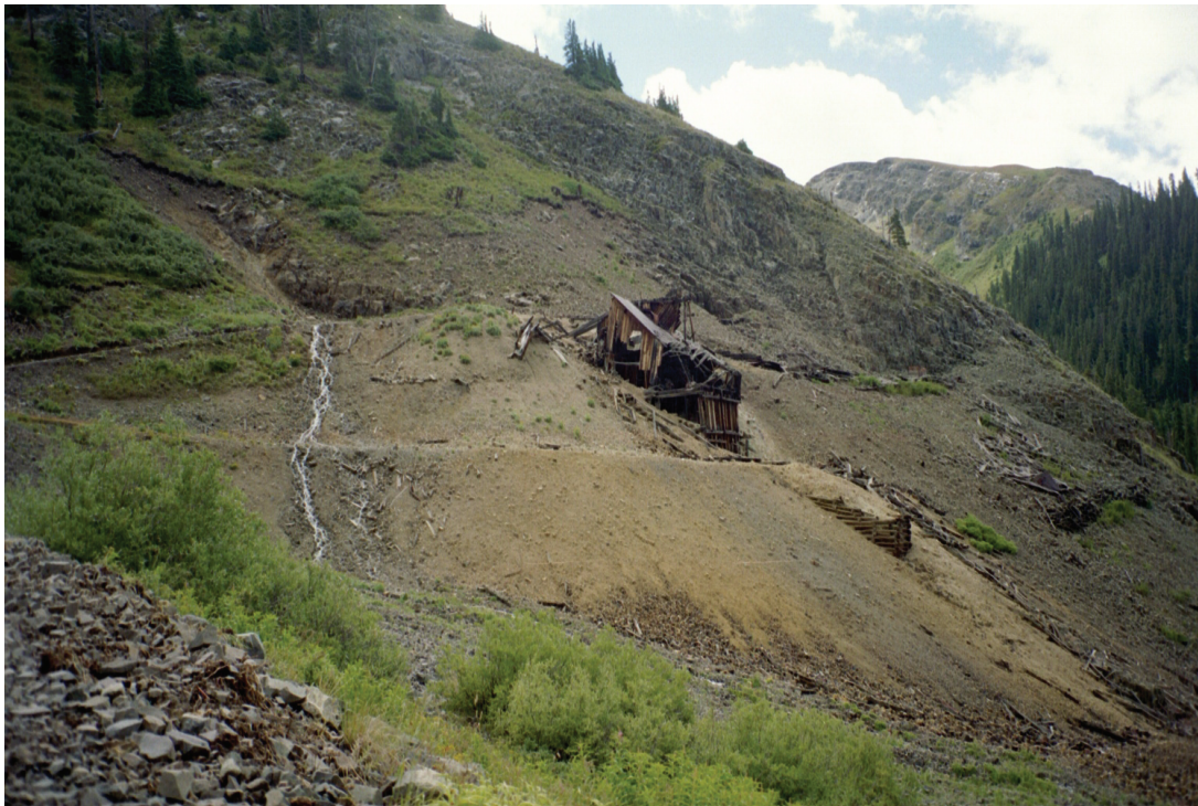
Figure 9. The Kittimack mine has a dump of modest size and relatively low sulfide content, but water flowing from the caved adit (left side of photo) is of concern. Although the pH of the water (5.8) is not highly acidic, the water carries substantial amounts of zinc.
