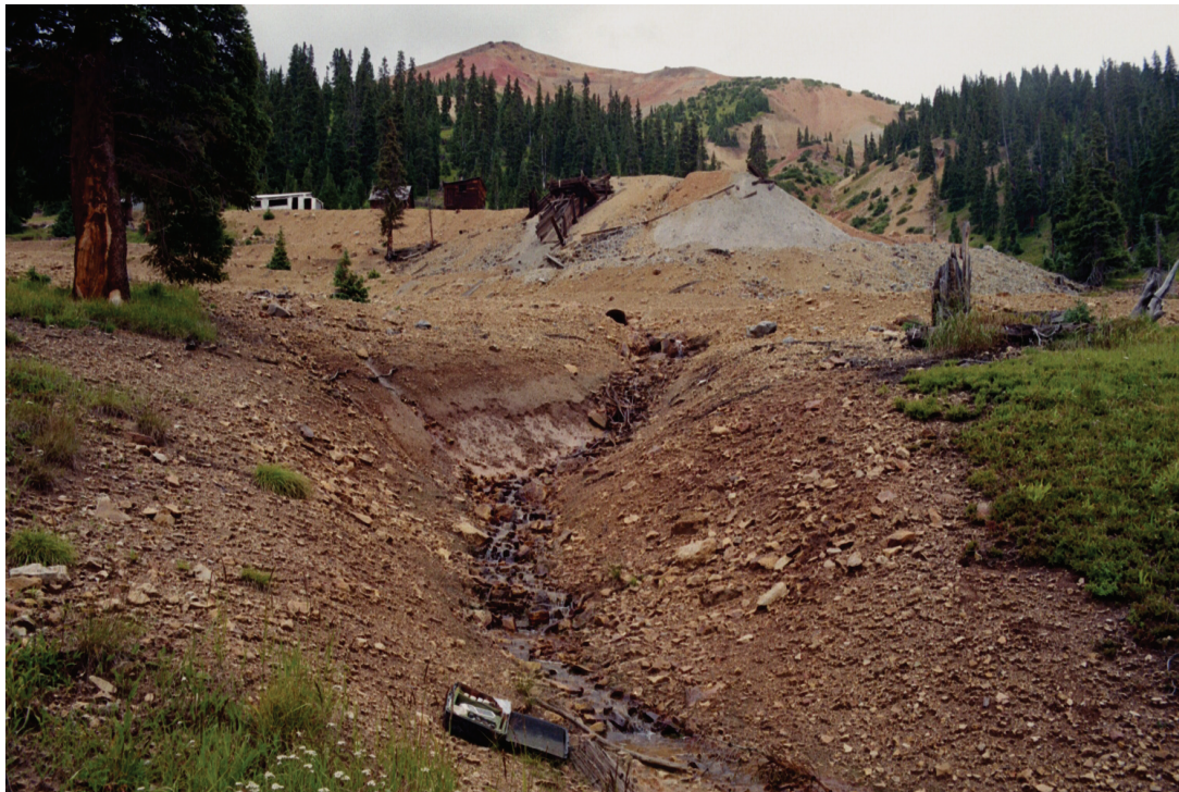
Figure 10. Lark mine on flank of Red Mountain # 3 created a dump of modest size but relatively high sulfide content; the dump was reclaimed by BLM in 2002. More complex are springs in the hillslope below the mine that are highly acidic and rich in metals; the springs are of uncertain origin despite several detailed studies.
