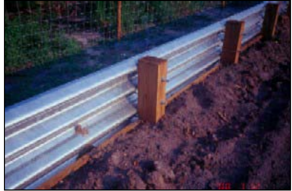
Type-A fence adjacent to southbound lane of U.S. 441.
