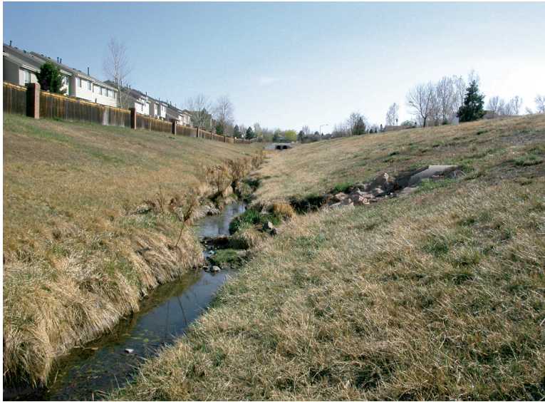
Figure 2. View of typical graded slope along bank of Toll Gate Creek.
