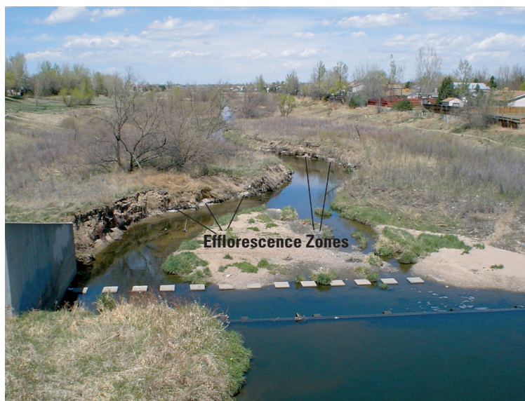
Figure 8. View of efflorescence zones along West Toll Gate Creek directly north of Mississippi Street overpass.
