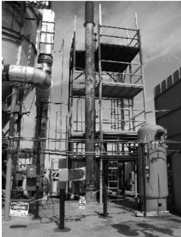
Figure 3-2. TEAD Incinerator Stack
