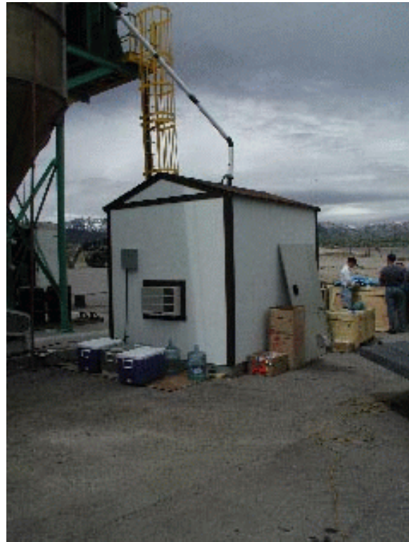
Figure 2-2. XCEM Housing and Gas Transport System at TEAD
