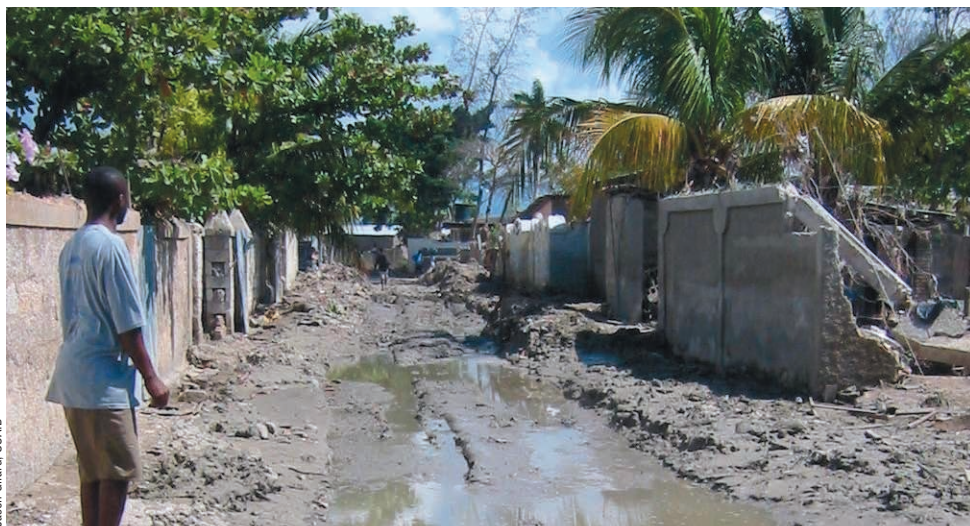
Though flood waters have receded in Gonaïves, Haiti, there are plenty of reminders of the damage from Tropical Storm Jeanne, including this mud-soaked roadway.
