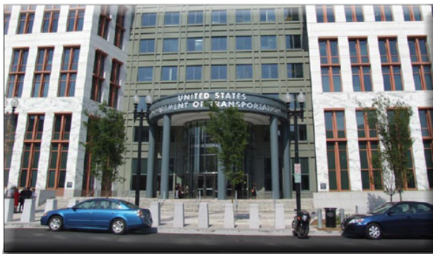
The Department of Transportation Headquarters.
