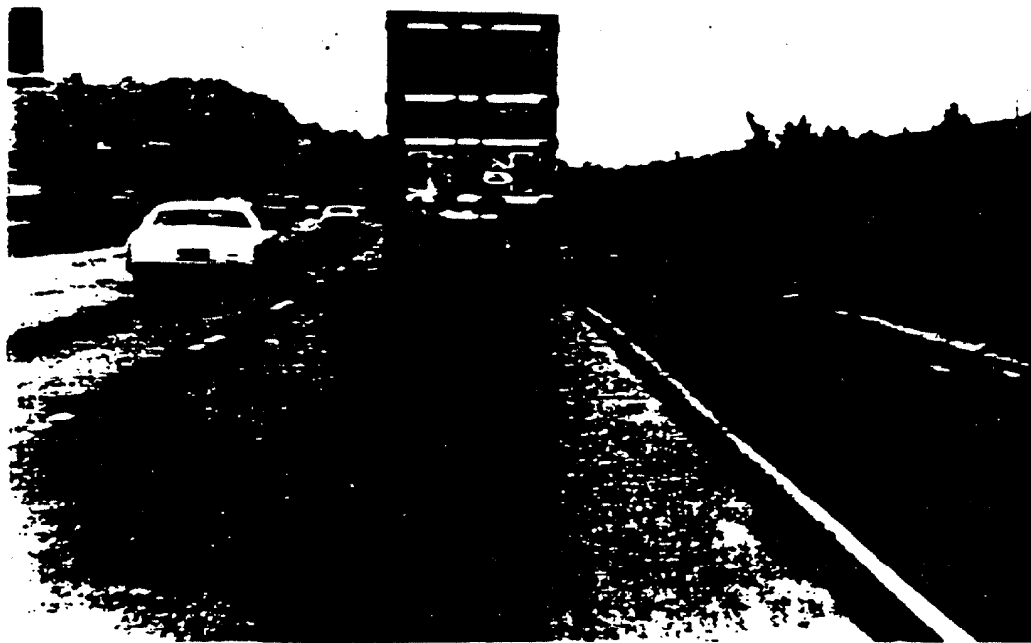
Photo 3 - A truck travelling near the edge of pavement. Note the pavement edge stripe location (12-ft PCC pavement slabs).
