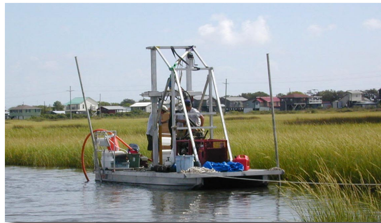
Auger system set up on an aluminum platform at Cocodrie, LA.
