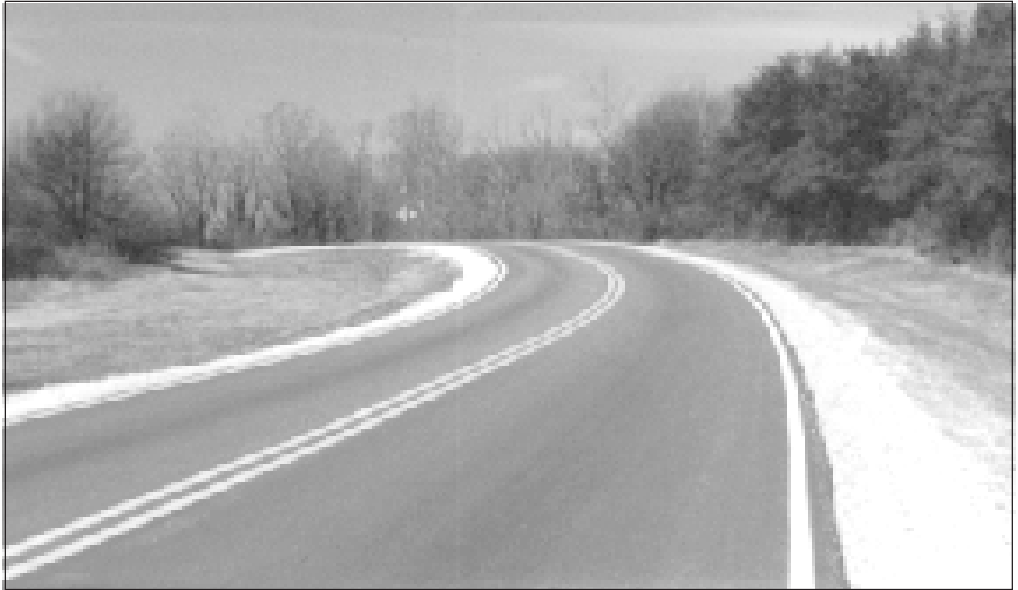
The end result of proper pavement preservation is a highway with an extended service life—thus saving funds—and a highway that provides a more consistent, better overall ride quality.
