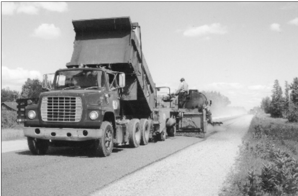
Michigan DOT relies on a wide variety of preventive maintenance treatments to extend the life of its pavements. Here, a chip seal is applied.
