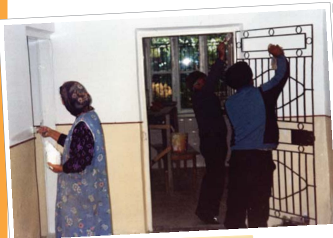
Community board volunteers rehabilitate day care center
