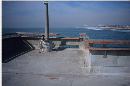
Figure 17-2. Scenic lookouts should provide a lowered viewing area for children, people who use wheelchairs, and people of short stature.
