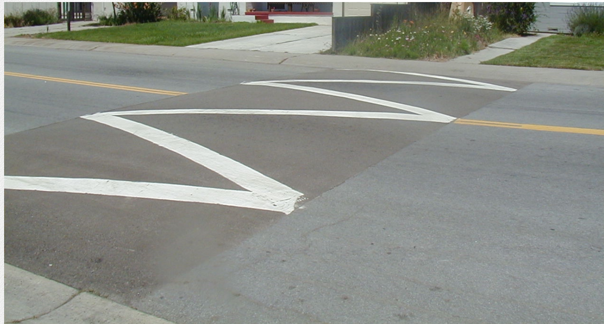
Figure 9-8. Speed humps are a common vertical measure for controlling the speed of motorists in residential neighborhoods.
