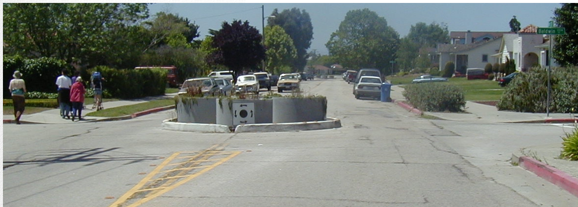
Figure 9-17. Neighborhood traffic circles are a common horizontal measure for controlling the speed of motorists at a low volume intersection.
