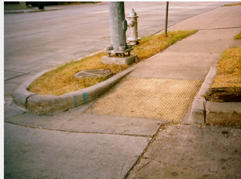
Figure 7-18. Detectable warnings at the bottom of curb ramps enhance access for people with vision impairments (Austin, Texas).
