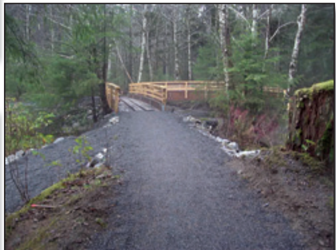
Figure 19—A finished trail bridge approach in the Tongass National Forest.
