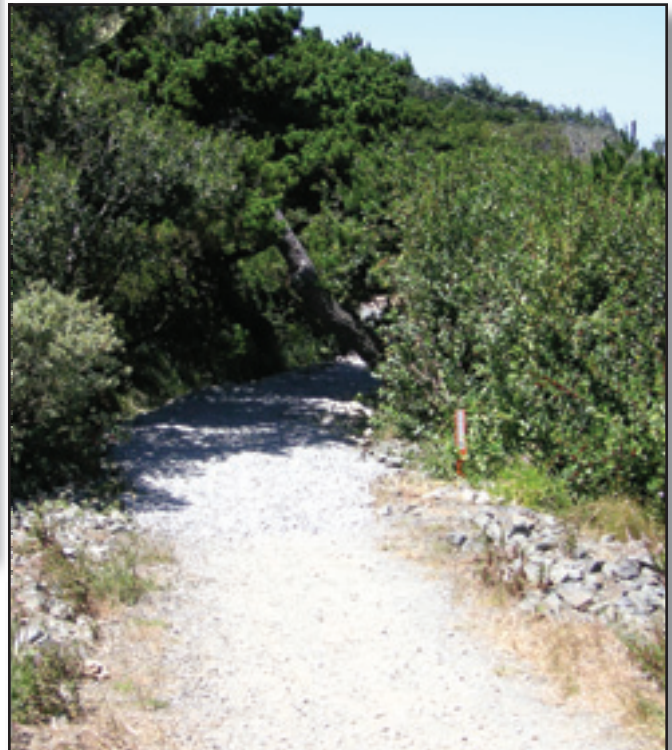
Figure 22 —A finished rock and geotextile underdrain.
