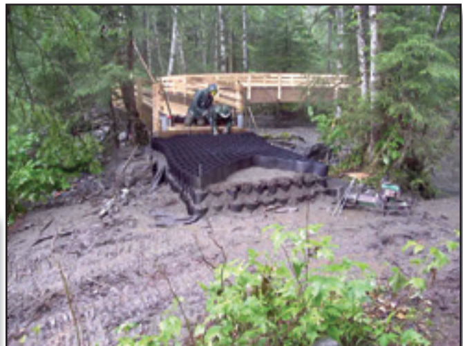
Figure 18—Using geocells to construct a trail bridge approach.
