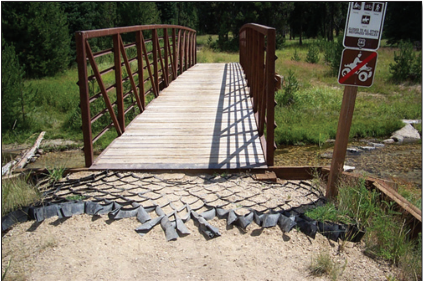
Figure 23—Geocells placed too close to the surface may unravel. The top of the geocell should be 2 to 3 inches below the surface of compacted tread fill.
