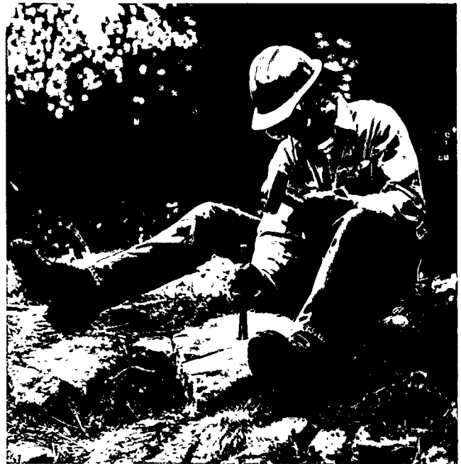
Single jack driller at work.
