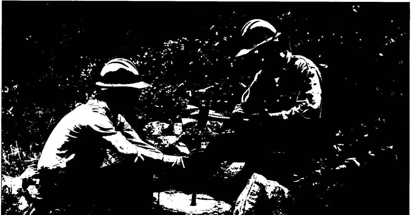
Modified double jacking team at work.
