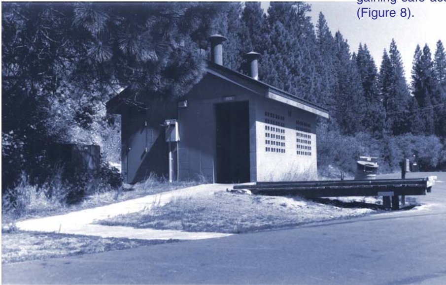
Figure 7—A timber boarding platform built alongside an existing restroom.
