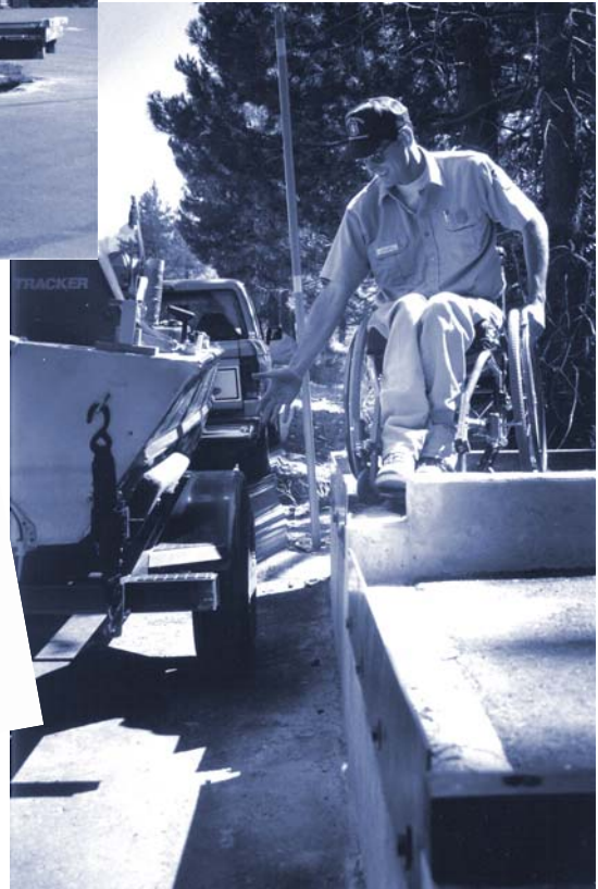
Figure 8—A ramp recessed behind curbs makes loading and unloading difficult.
