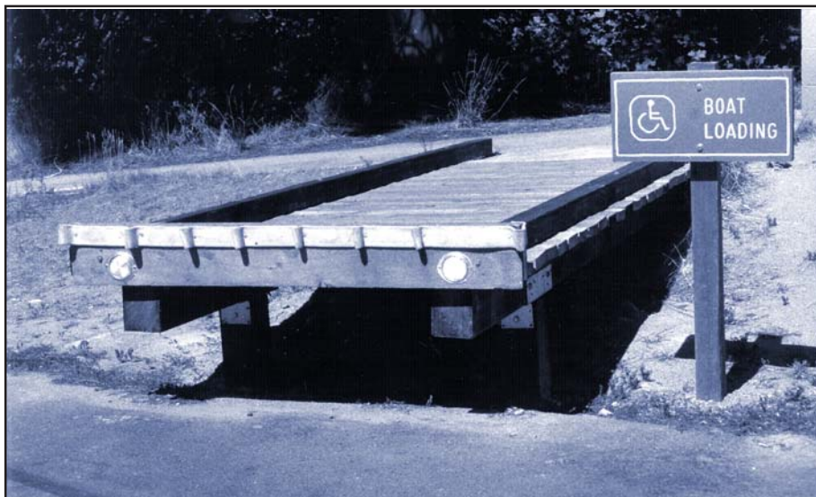
Figure 4—A typical timber ramp.
