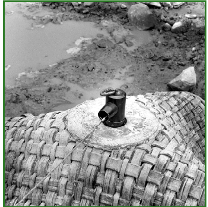
Figure 10—The lanyard is attached to the firing mechanism.
