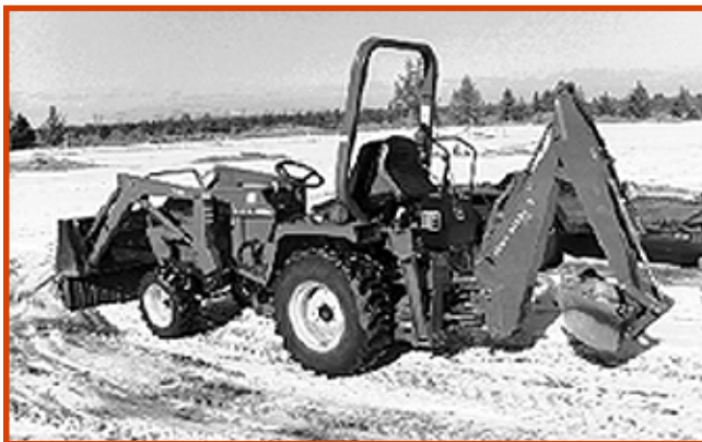
Figure 22—Utility tractors are very versatile and useful for heavy-duty trail work.
