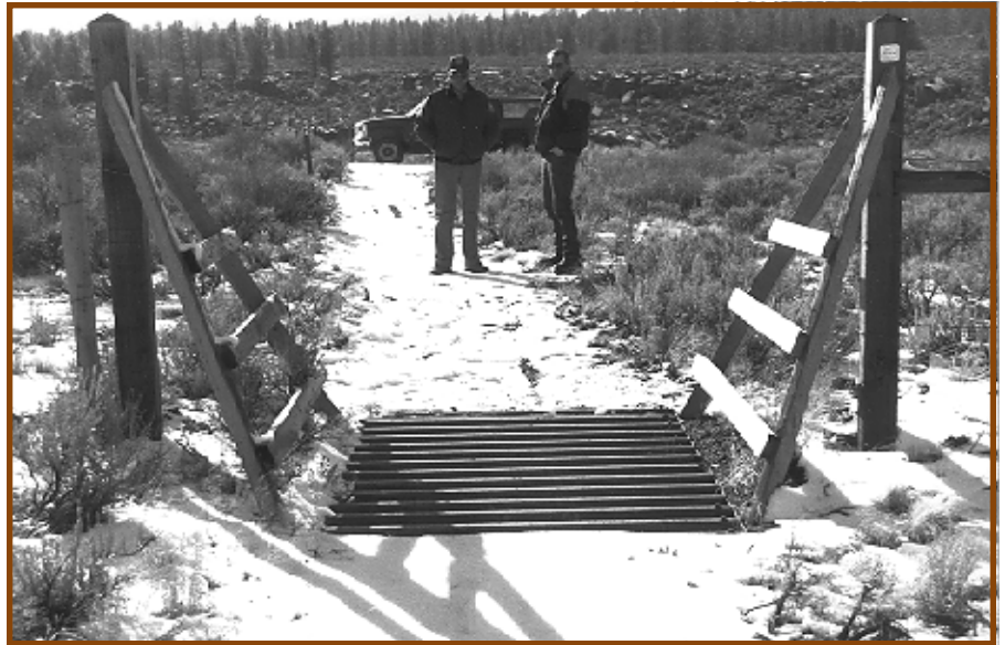
Figure 4—The Deschutes Trail Cattle Guard looks and performs like a downsized version of a traditional road cattle guard.
