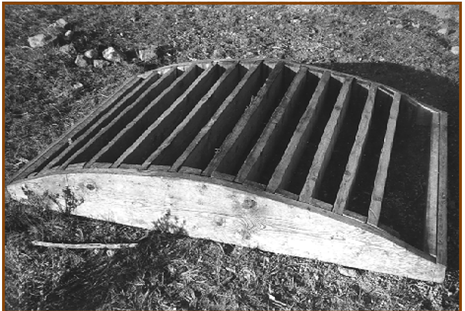
Figure 8—The Challis Trail Cattle Guard. Treated 2 by 6's are used for tread rails. (One piece of decking is missing on the right side.)
