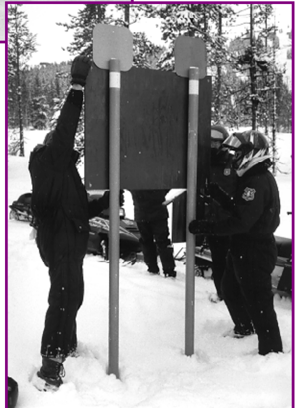
Figure 13—ReflectORIZED tape greatly improves the sign's visibility at night.
