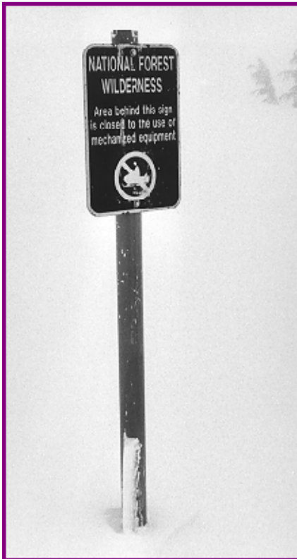
Figure 10—PVC pipe has worked best to post the Three Sisters Wilderness boundary. The upper two-thirds of the pipe is painted orange to improve visibility.
