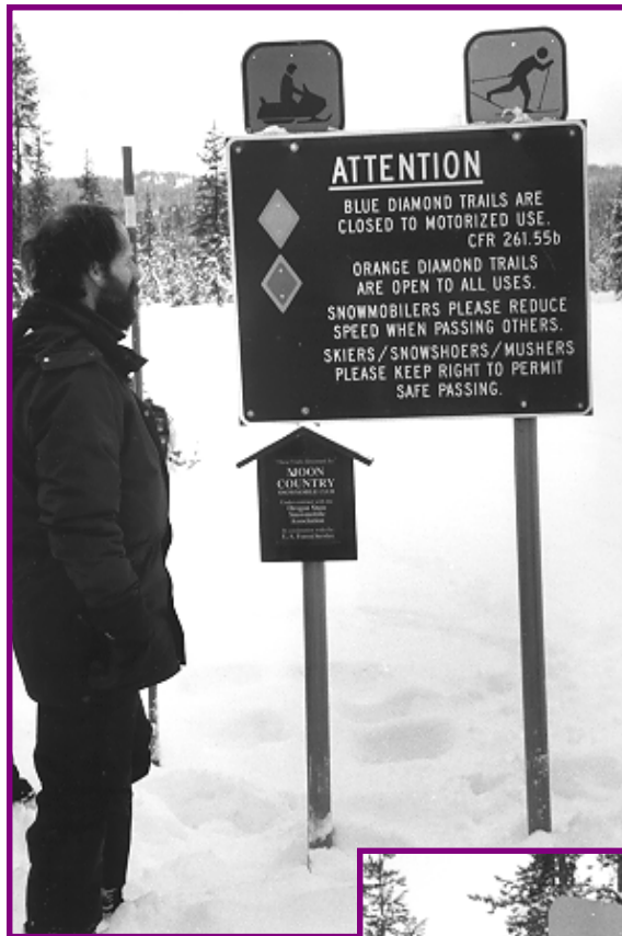
Figure 12—Two PVC pipes hold this large sign in place. Because the posts are not anchored to the ground, they can be raised as the snow becomes deeper.
