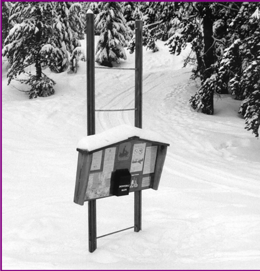
Figure 7—Simplicity itself. Hooks on the back allow the bulletin board to be moved from one rung to the next. Hooks are much easier to work with than nuts and bolts. Two people can easily lift the bulletin board to the next rung. Supplemental security bolts or a lock and chain could be added in areas where users tend to evaluate signage by its warming fire potential.
