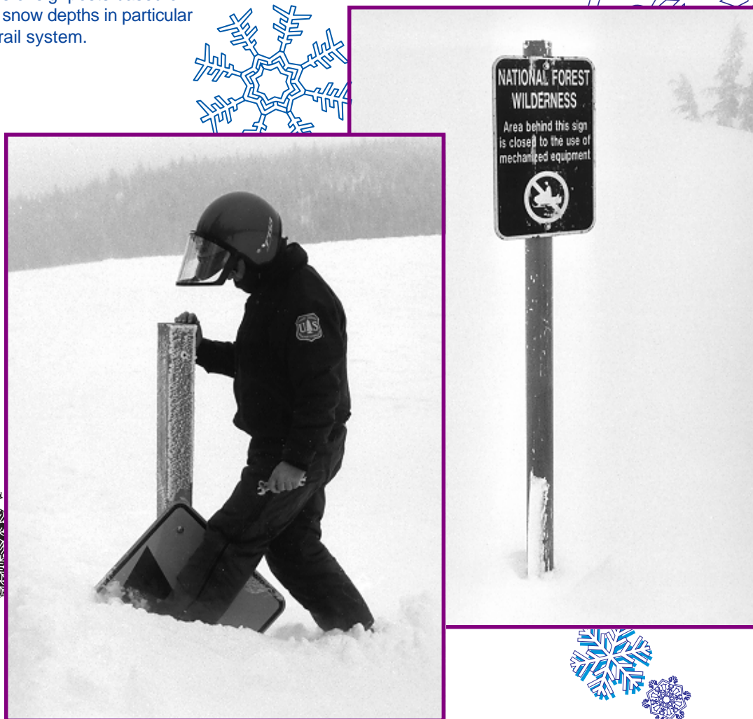
Figure 3—Minus zero: Icy nuts dropping into the snow. Signposts frozen in solid. High winds and poor visibility. Oops! There goes the wrench! Good reasons to keep your signpost system simple.
