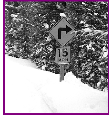
Figure 5—AFTER: Raising the sign to a higher set of holes makes it effective once again. Some Districts use permanently set signposts up to 16 feet (4.9 m) tall with holes drilled at several levels.
