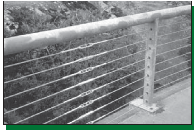
Figure 63—Wire rope is used here as part of the railing system.
