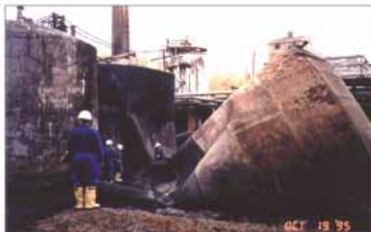
C. Tank 488, after explosion.
