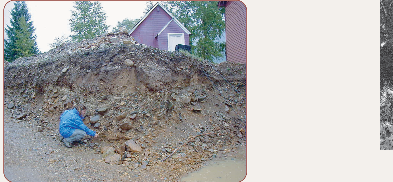
Figure 8. Alluvial ferricrete at base of excavated foundation (town of Silverton). Builders commonly encounter ferricrete "hardpan" when excavating foundations throughout the town.
