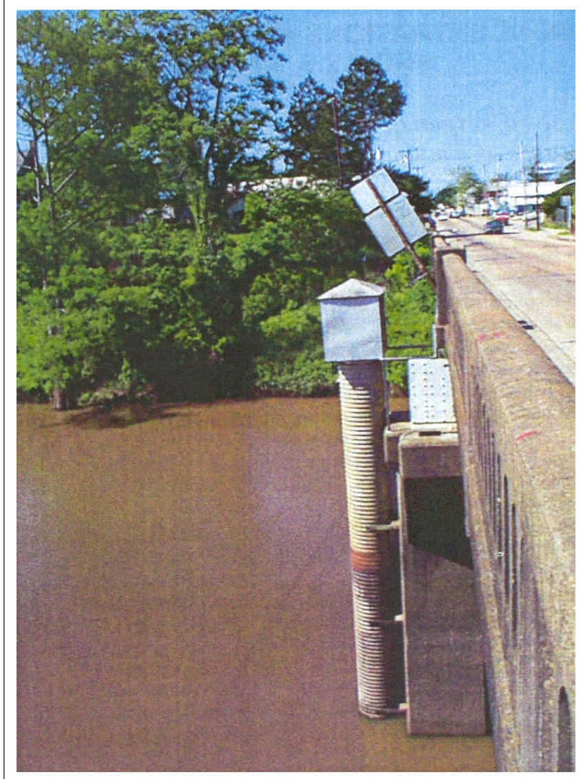
Figure 2.2-1. Water-quality data-collection site at Bayou Courtableau at Washington, Louisiana. (Photograph by Todd E. Bauman, U.S. Geological Survey.)
