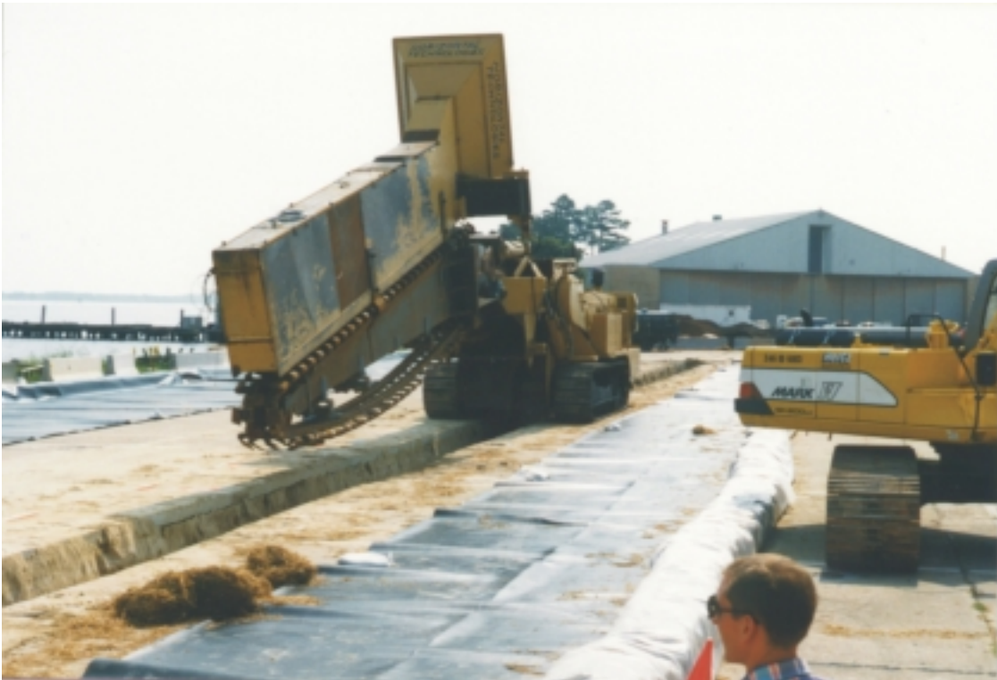
Figure 54. Plastic sheets laid down around trench for erosion control.
