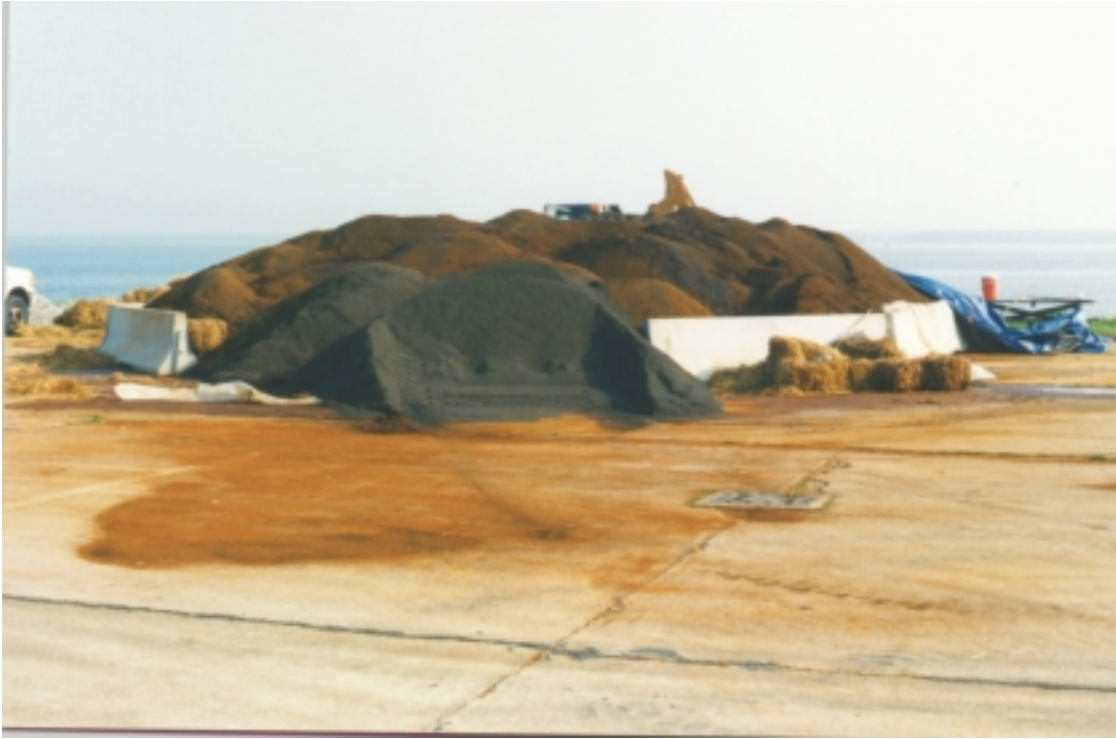
Figure 53. Peerless™ iron filings stored on site.
