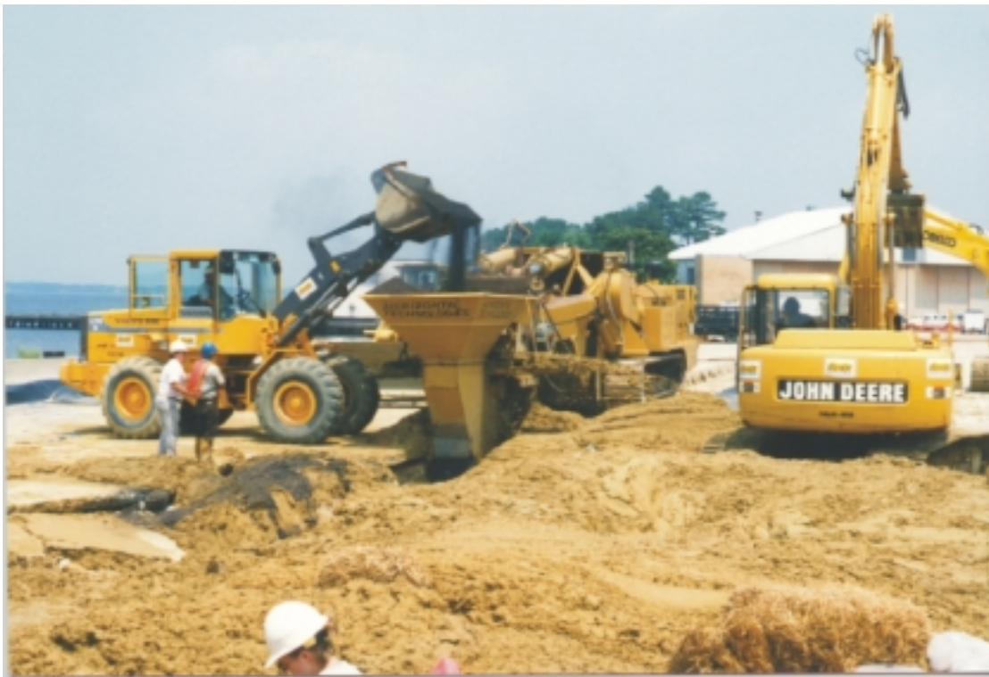
Figure 56. Excavated aquifer sediments on either side of the trench.
