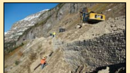
Mechanically stabilized earthen wall - FHW photo
