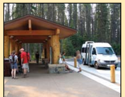
The new Apgar Transit Center - David Restivo photo
