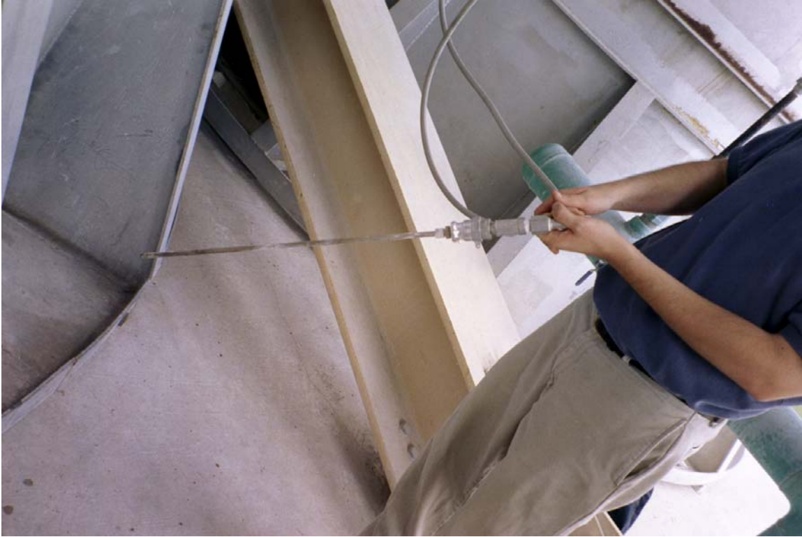
Figure 8-9. Suwannee American Cement ammonia injection nozzle.
