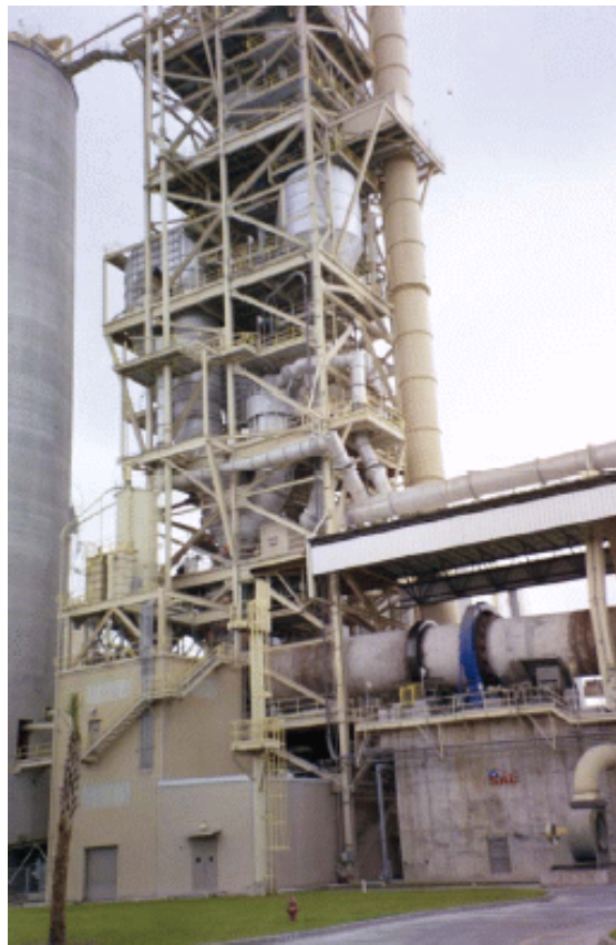
Figure 3-4. PH/PC kiln system.
