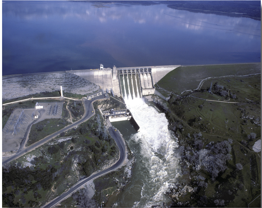
Folsom Dam (photo courtesy of USBR)
