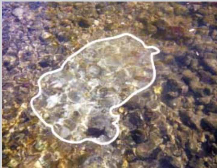
Scour hole downstream from P4 (upstream from TS4), about 5.5 feet wide.
