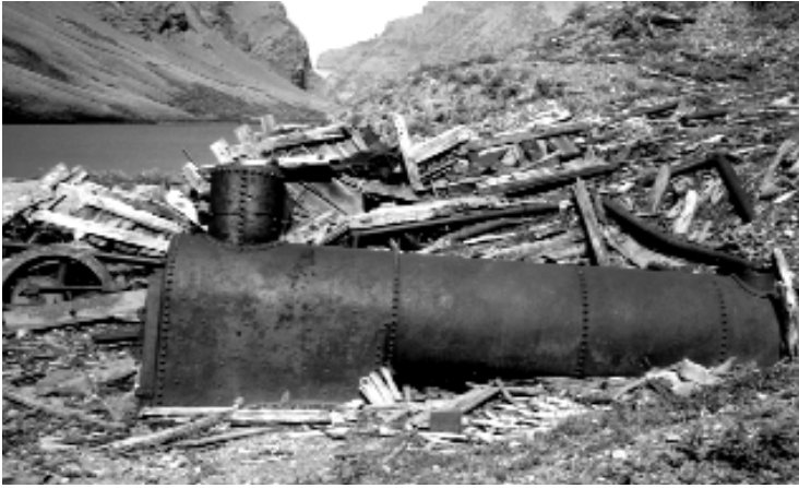
Close-up of Cracker Mill boiler with lake in background
