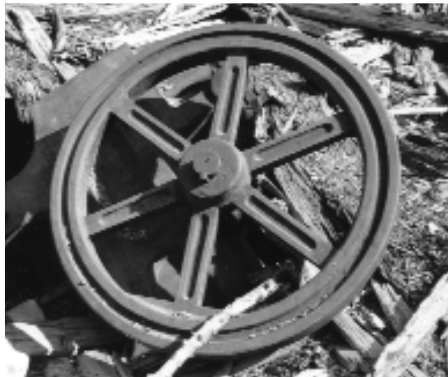
Collapsed Cracker Mill and bull wheel.
