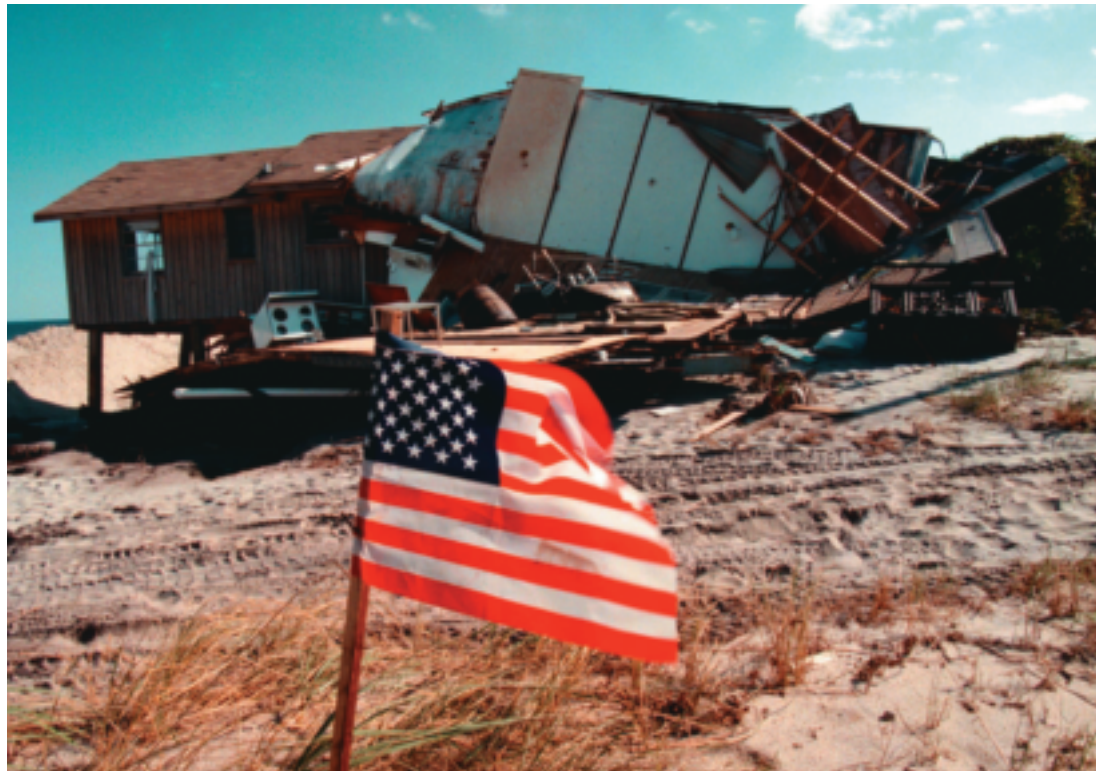
Aftermath of Hurricane Fran, September 1996, Photograph by Dave Gatley, from FEMA Photo Library
