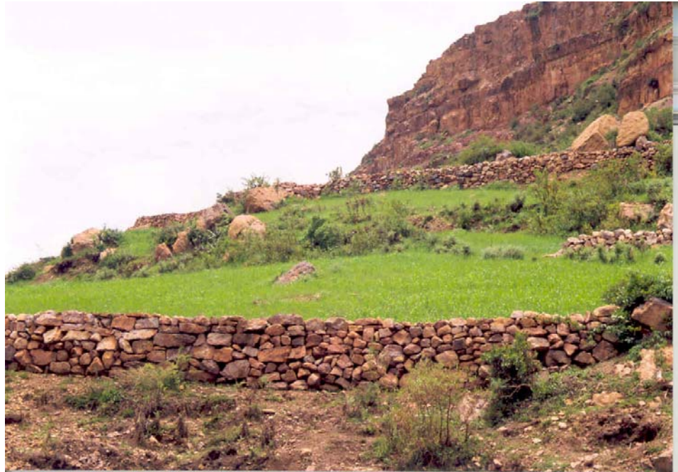
Photograph of stone bunds, one of the projects built by the beneficiaries of REST's food for work program in Degua Tembien, Ethiopia. Stone bunds prevent soil erosion. (August 2003)
