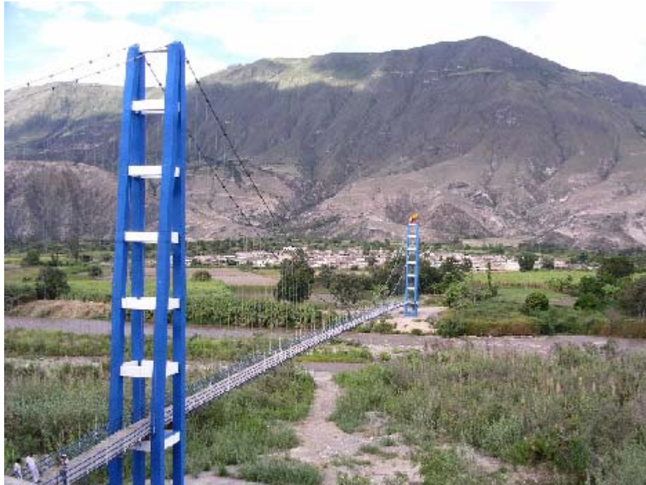
Photograph of Chota River pedestrian bridge in the Province of Carchi taken in June 2004.
