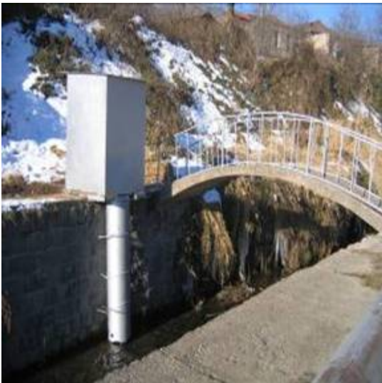
Photograph of a water monitoring station rehabilitated by the USAID-funded Water Development Project, March 2007.
