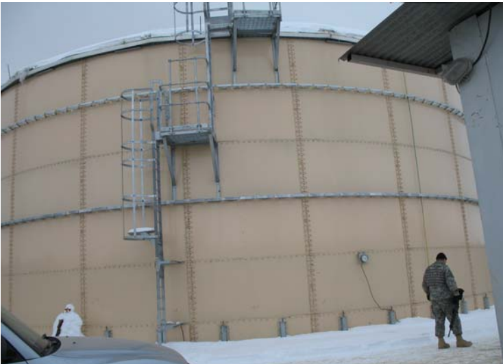
OIG photograph of a USAID-funded steel reservoir used to hold water from production wells before being sent through the water distribution system. Gardez, Afghanistan (December 2006)
