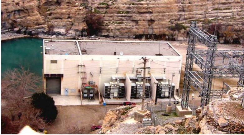
OIG photograph of the Kajakai Dam power plant located at the toe of the Kajakai Dam and bank of the Helmand River. (January 2007)
