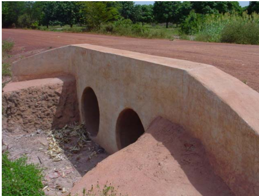
Picture of a water conduit constructed with SSH funds in the Koulikoro region of Mali on October 22, 2002.
