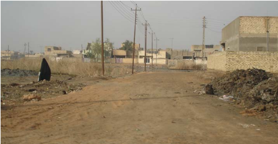
Photo of a road repaired through an OTI/Iraq grant. (South Central Iraq, February 2006)
