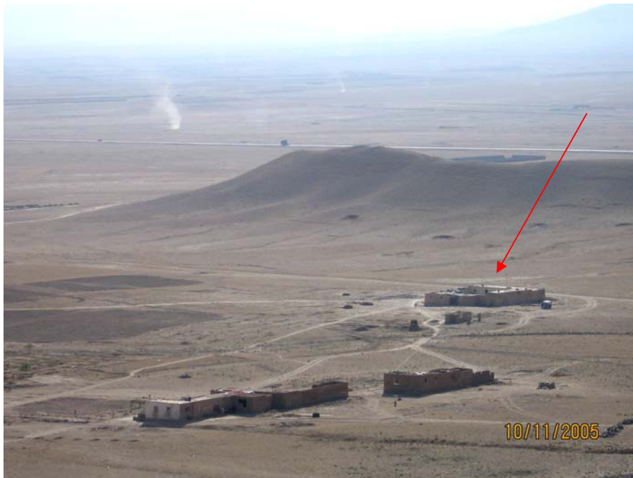
Photograph taken October 11, 2005 by an OIG auditor of the compound—identified by the red arrow—located on the Chil Dukhtaran housing development site.
