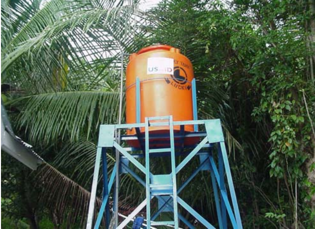
OIG photograph of a USAID-supplied water tank used to improve the water supply to a village health clinic in Desa Nusa, Aceh Besar District (Aceh Province, Indonesia, February 2006)
