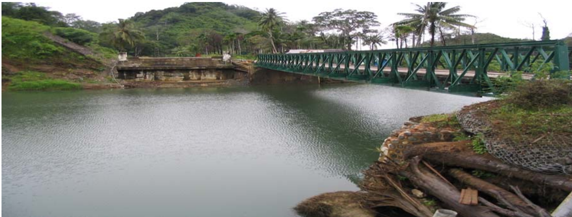
OIG photograph showing all debris had been removed from a bridge that was destroyed by the tsunami. Remnants of the bridge can be seen on each bank just left of the new temporary bridge. (Aceh Province, Indonesia, November 2005)
