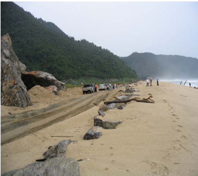
OIG photograph of a section of the Banda Aceh-Lamno road where the original road was destroyed by the tsunami and a temporary dirt road was put in its place. (Aceh Province, Indonesia, November 2005)
