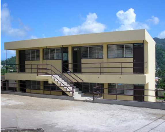
Photo taken on January 19, 2006 by an OIG auditor of a newly constructed school (Happy Hills) financed by USAID/Jamaica in Grenada. The school was open and operational on January 1, 2006.
