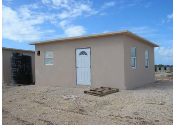
Photo taken on January 13, 2006 by an OIG auditor of a house built by the ONR in Jamaica.
