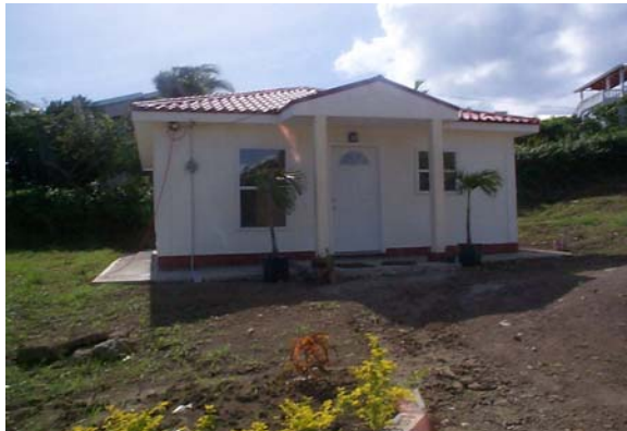
Photo taken by The Housing Authority in December, 2005, of a 510 square foot steel frame house with a tile panel roofing system. This house was built during the hurricane reconstruction period for resale to the public in Grenada.
