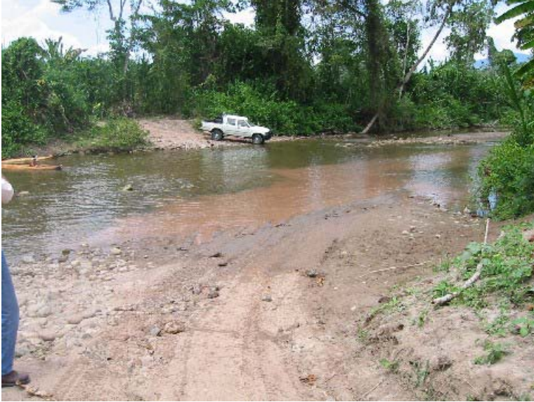
Photograph taken by an OIG auditor on September 1, 2005 of a stream that cuts across a road that was rehabilitated under the ADP program, rendering it impassable during the rainy season, in Chazuta, Peru.
